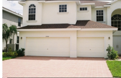
Acceptable: upper floor pushed back from front of garage.
