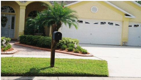
Unacceptable installation: paver material not flush with curb and street sidewalk. The paver material itself is acceptable.
