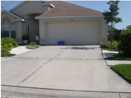
Unacceptable: driveway extension on right hand side is in excess of 2ft
