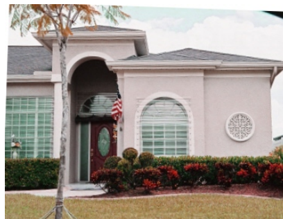
Unacceptable: plastic panels permanently attached to home.
