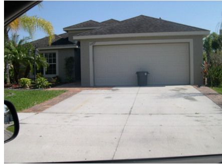
Unacceptable paving extending into driveway
