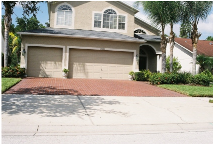
Two different materials for driveway and walkway is acceptable as long as one of them is concrete and the other is pavers.
