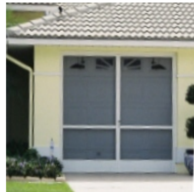
Unacceptable: screened in over garage door
