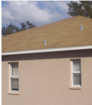
Acceptable: Minimum 30-year asphalt dimensional shingle
