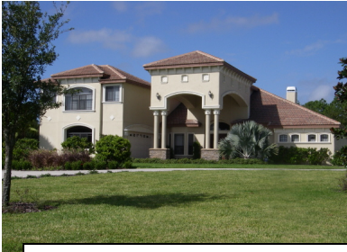
Unacceptable: entry and garage out of proportion to rest of house
