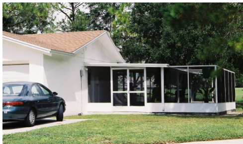
Unacceptable: prefabricated screen room.
