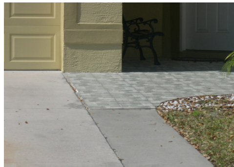
Acceptable: entryway and extension are different applications however driveway extension is concrete
