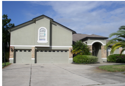
Unacceptable: "lopsided" upper floor on one side
