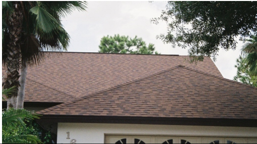
Acceptable: Minimum 30-year asphalt dimensional shingle
